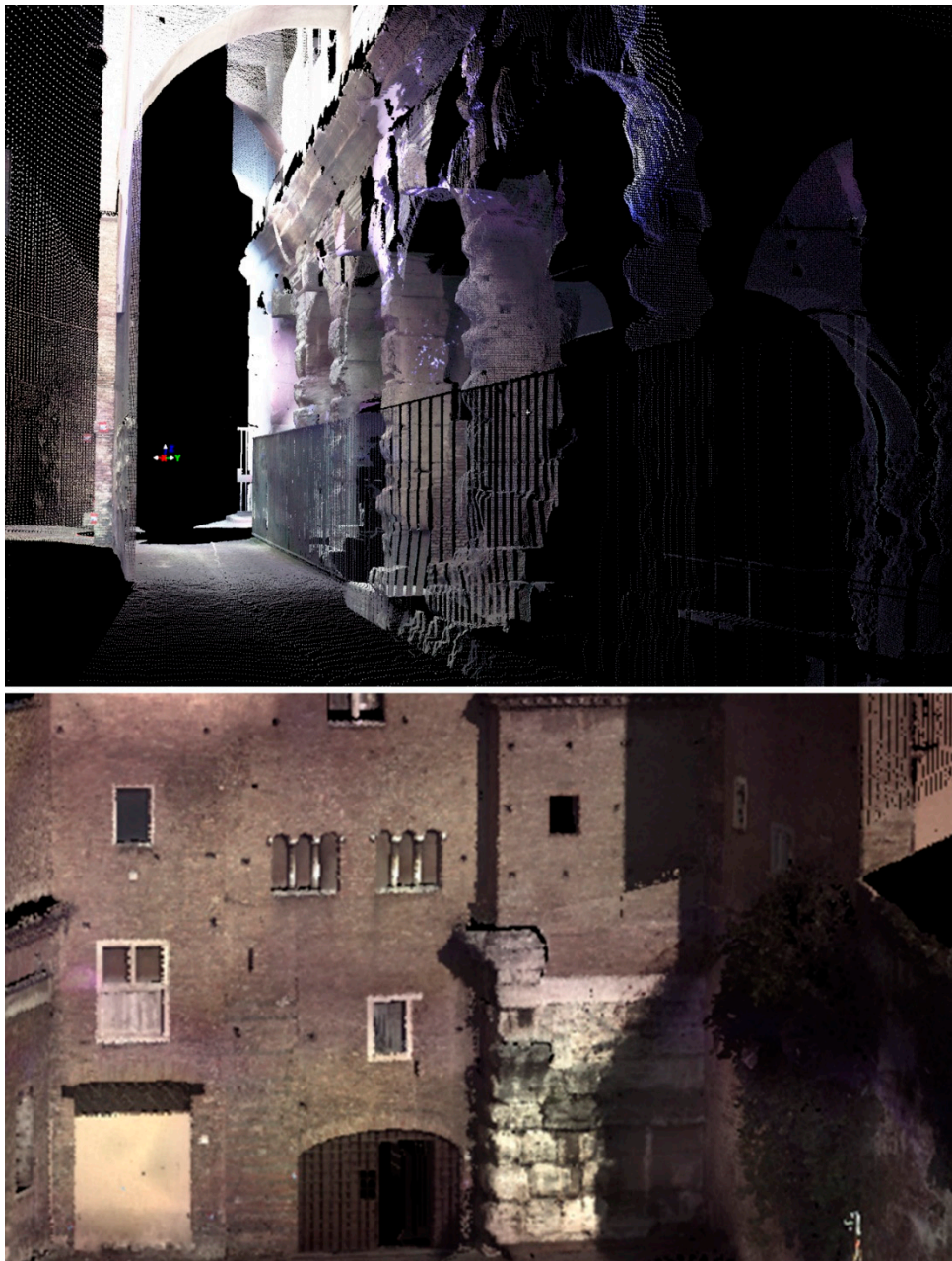
Figure 4. The Temple of divo Claudio. Views of the numerical mode RGB reflectance and RGB color.
