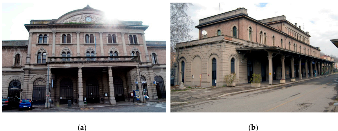
Figure 2. Picture of Piazza Manzoni Station: (a) main façade and (b) secondary façade with shelter.
