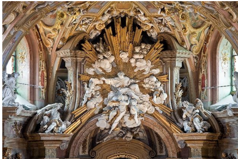
Figure 4. Stucco decoration in the Holy Hill near Olomouc, image before restoration works.
