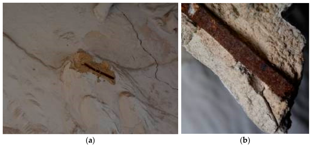
Figure 2. Heissler's study room: (a) broken eagle's head; (b) the close-up image shows the internal structure. The ground mortar (sample JUHE 002) is wrapped around a squared iron bar app. 10 mm × 6 mm across and finished with a stucco finishing layer (sample SUHE 002).
