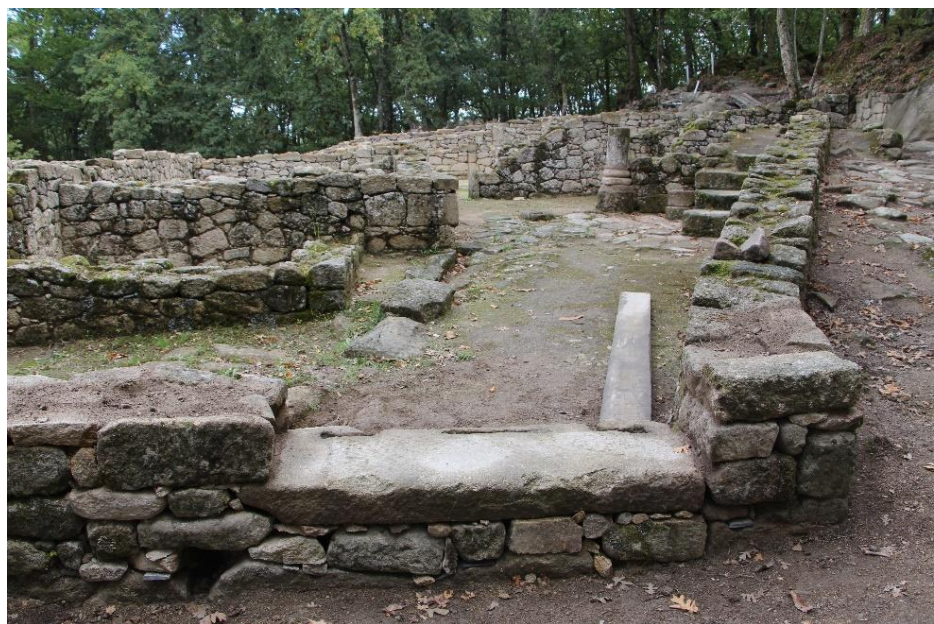
Figure 20. Final view of the area after the opening of the entranceway and the installation of the threshold.
