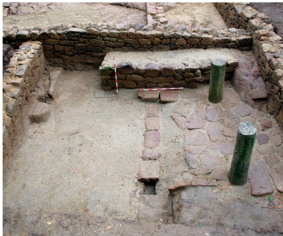
Figure 11. Final state of the atrium after the restoration works in 2014. Photograph: David Pérez.
