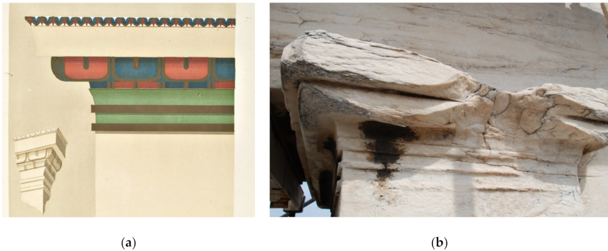
Figure 18. (a) Impost block of the central building of the Propylaea (coloured drawing, Penrose. pl. 26 [29]). (b) Impost block of the north-west anta, south side, macroscopic view. A red paint layer is visible underneath the black crust on the Doric cyma (red frame). A green paint layer is preserved underneath the black crust on the interval between the second and the third annulet (from the bottom to the top).
