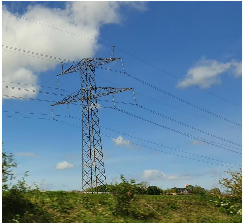
Figure 11. Dominant power lines at house in Denmark. Photo: Vandrup Martens.
