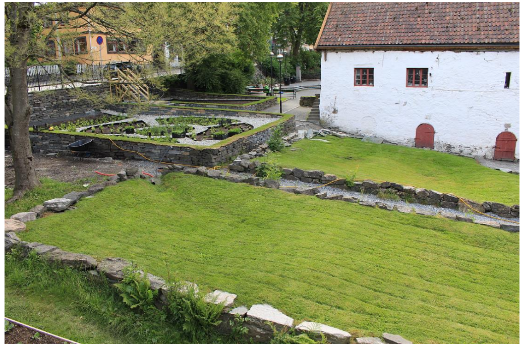
Figure 15. Rainwater bed and infiltration bed at Bryggen in Bergen, Norway. Photo: Dunlop, NIKU.
