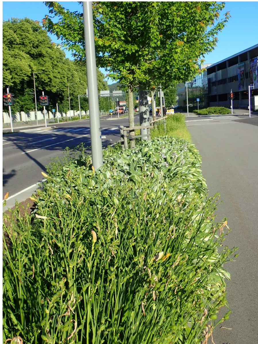
Figure 13. Rainwater beds along a busy street in Drammen, Norway. Photo: Vandrup Martens, NIKU.
