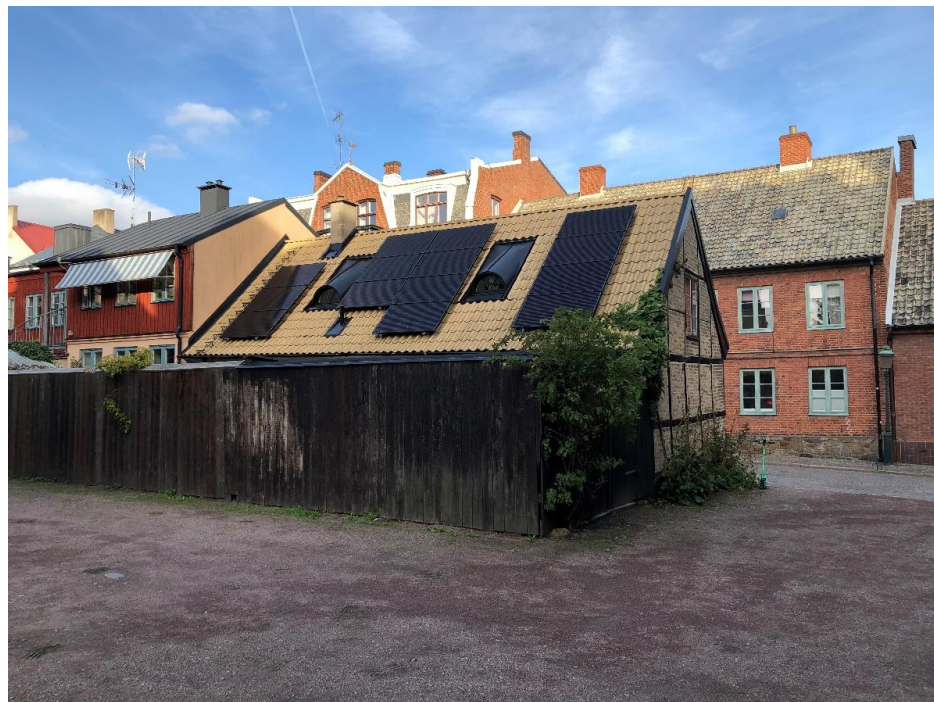
Figure 2. Solar panels on roof of historic building, Lund, Sweden. Photo: Haugen, NIKU.
