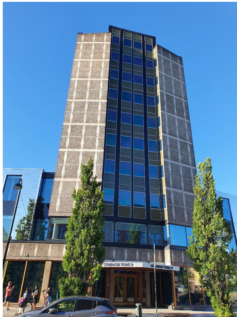
Figure 4. Solar panels on modernistic building in Drammen, Norway. Photo: Vandrup Martens, NIKU.
