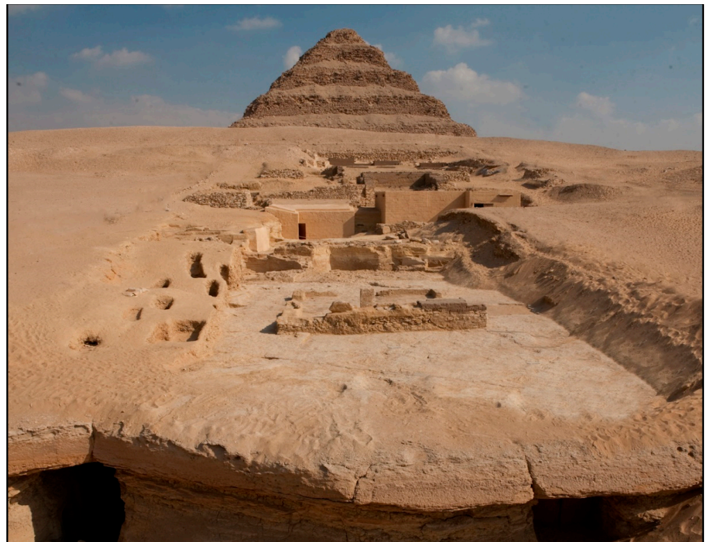
Figure 6. The late Old Kingdom cemetery west of the Step Pyramid complex—view from the west (phot. J. Dąbrowski/PCMA UW).
