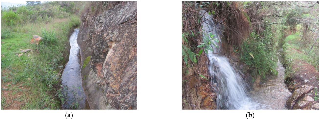
Figure 5. (a) Photos of the Spanish Canal along the base of the Cerro Morro Negro foothill just north of where water enters the Terrace Platform Complex; (b) a principle water fall for the Spanish Canal close to the diversion channel for the Molino la Mesopotamia.
