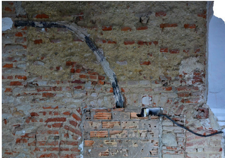
Figure S17. Detail of the factory of facing 4 of the original building; and basket-handle arch of the door of this facing
