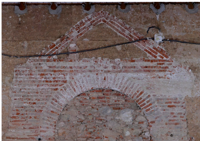
Figure S9. Detail of the front and the semicircular arch of the new open portal on facing 2
