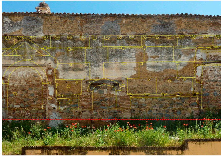
Figure S8. North facing 2, with the elements of the south face, georeferenced and indicating the original floor level of the cloister
