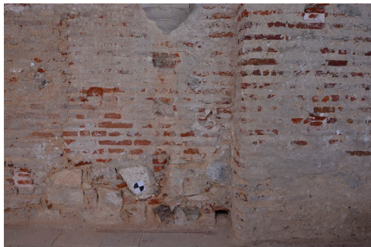
Figure S2. Detail of the facing of the church, the original wall and the reforms of the Cloister
