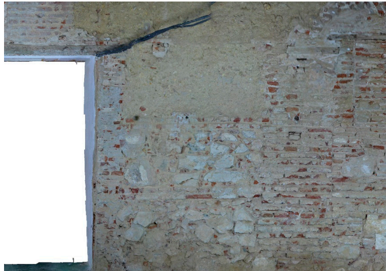
Figure S13. Detail of the masonry plinth and rammed earth wall of facing 3 of the original building
