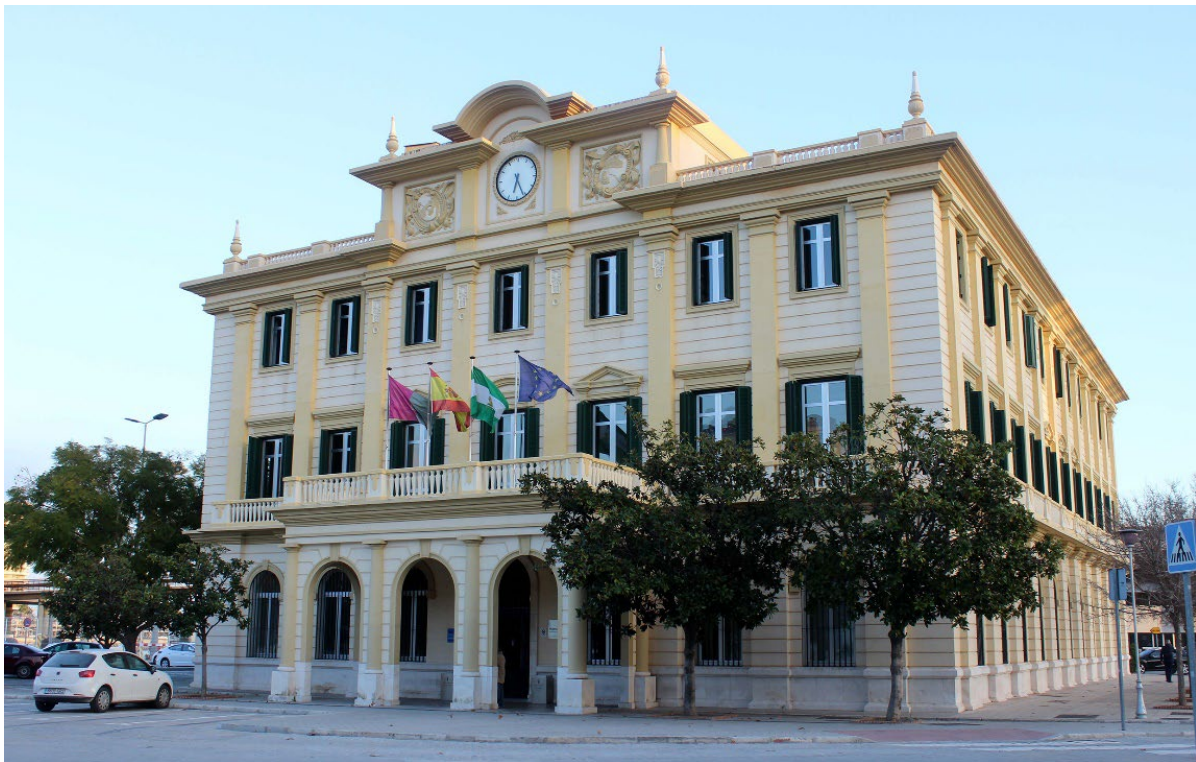
Figure 8. Port Board of Works, Malaga, Spain.
