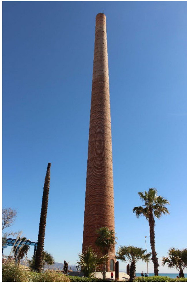
Figure 14. Los Guindos lead smelting factory chimney's, Malaga, Spain.
