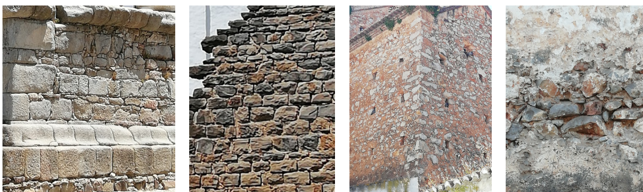
Figure 2. Identification of material: regular stones and cement plaster.
