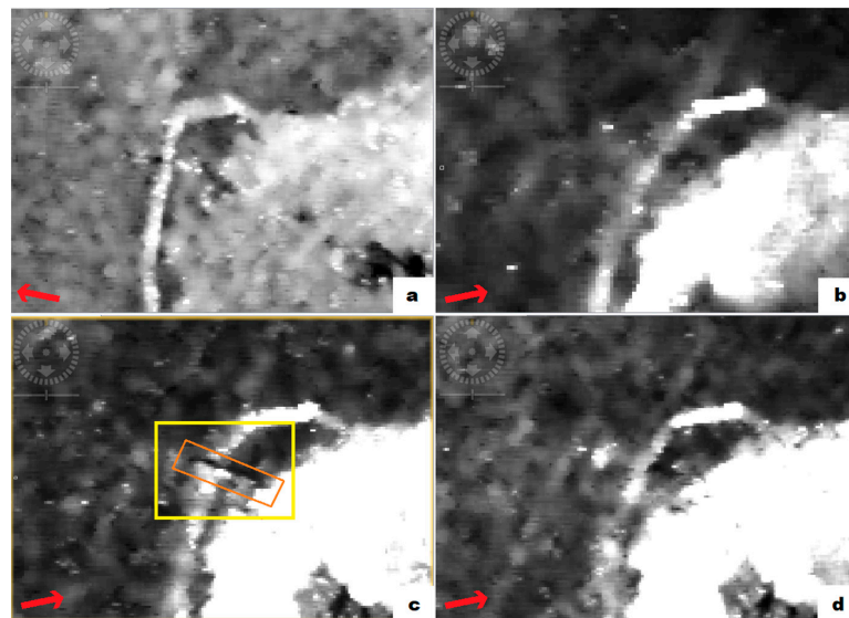
Figure 26. Filtered SAR images of the collapsed column. The yellow polygon in image (c) indicates the area where the column is, orange polygon shows the collapsed column and red arrow indicate the viewing direction of the sensor (SAR Acquisition dates; (a) 12 March 2023, Incidence angle center: 44.26^\circ , (b) 21 April 2023, Incidence angle center: 27.49^\circ , (c) 26 April 2023, Incidence angle center: 43.16^\circ , (d) 7 April 2023, Incidence angle center: 43.16^\circ —© DLR, 2023).
