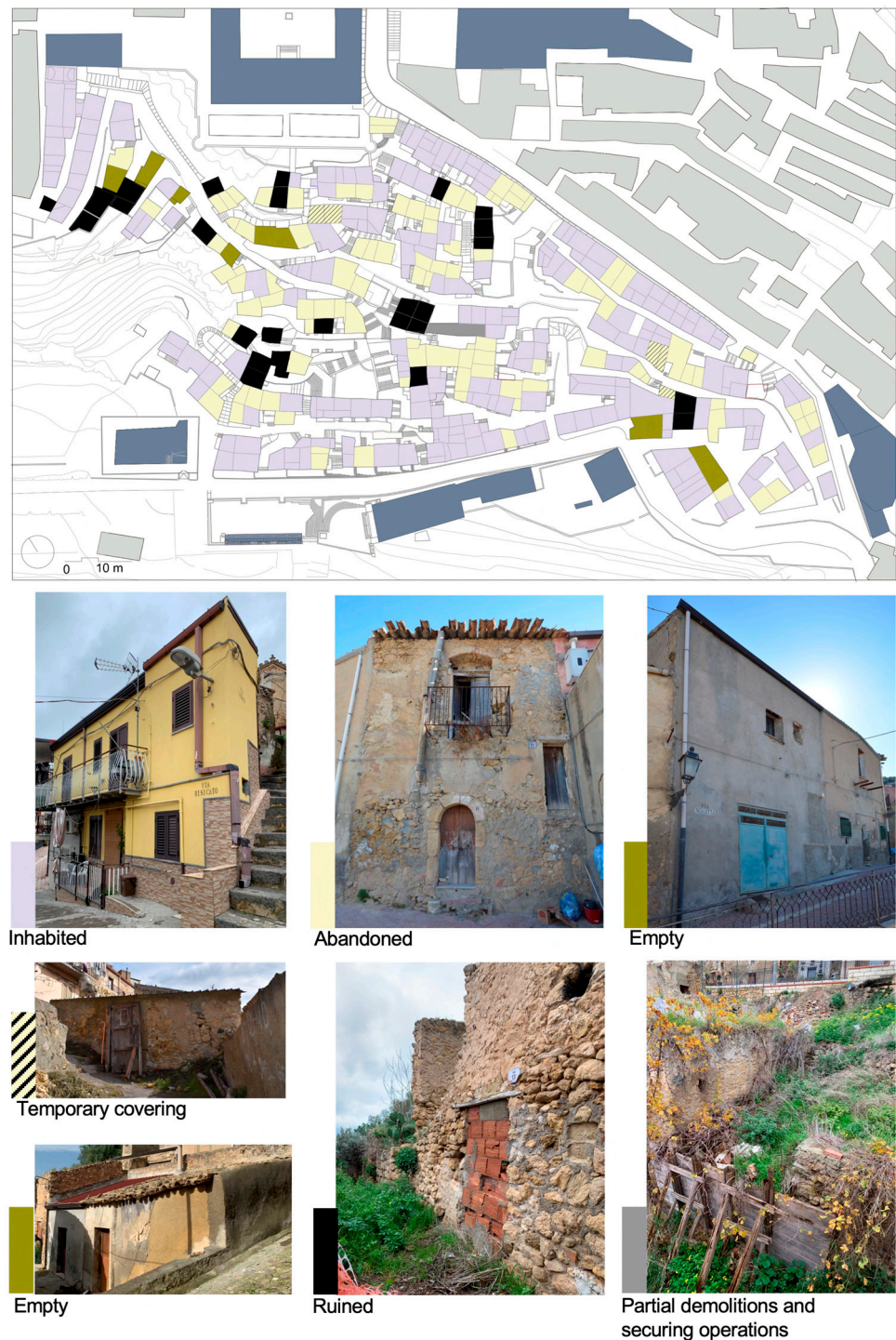
Figure 5. Survey of buildings according to their use and state of conservation. The analysis reveals a lack of homogeneity of conditions in the historic neighbourhood (our elaboration).
