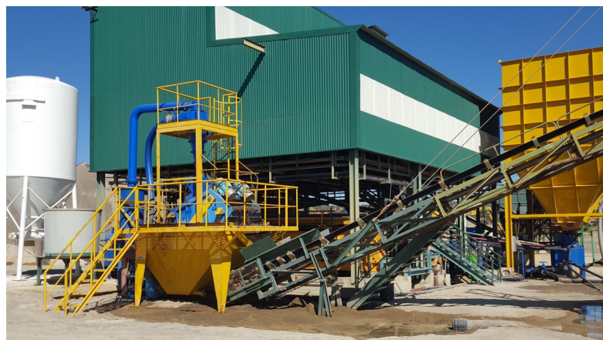
Figure 6. Infrastructure for recovering tungsten from waste and tailings in La Parrilla (Extremadura, Spain). Picture taken by D. Pereira.
