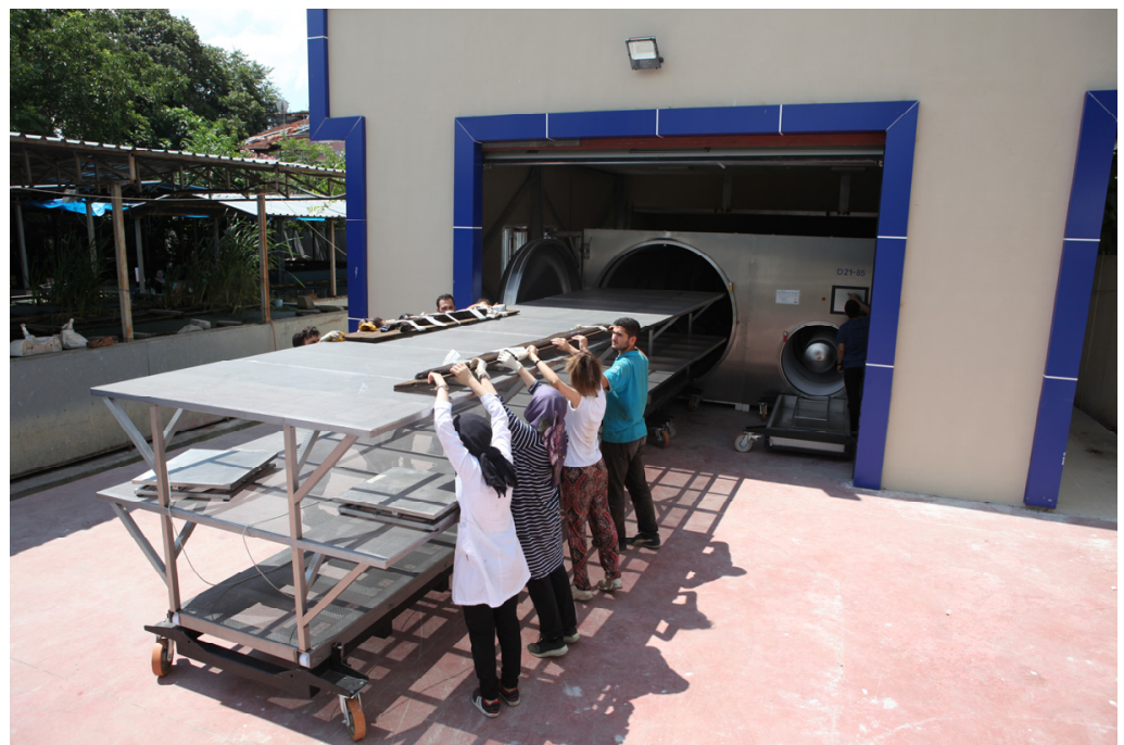
Figure 18. Vacuum freeze-drying device at Yenikapı laboratory ( \varnothing 2.10 m/L. 8.50 m). © YSP Archive.
