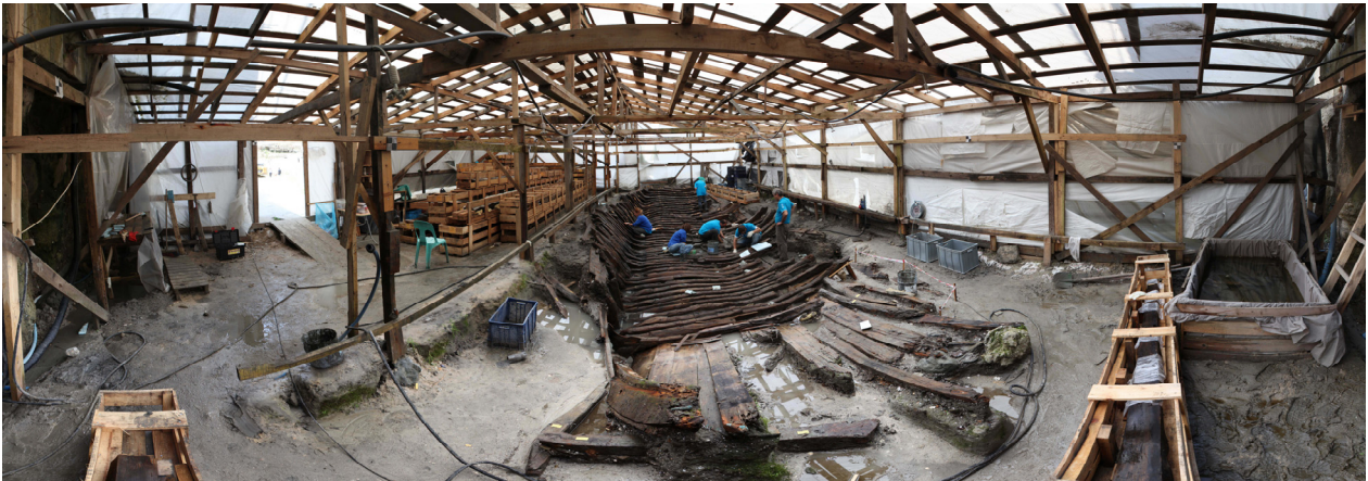
Figure 6. Dismantling process of shipwreck YK35's timbers. © YSP Archive.
