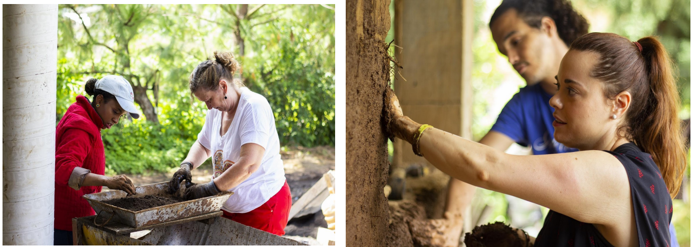
Figure 7. Preparation and application of the earthen refurbishments. Source: A. Solís-Sánchez.
