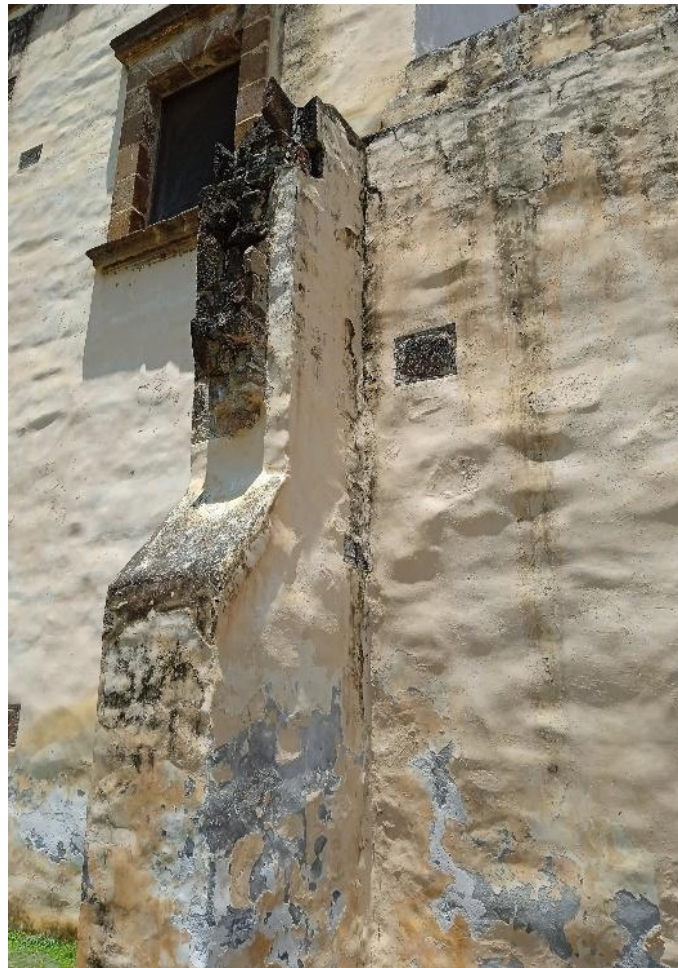
Figure 1. Pathology in contemporary cladding on a historical building in Patzcuaro, Michoacan, Mexico. Source: B. González-Sánchez.
