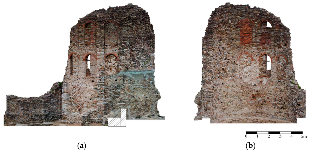
Figure 5. Church of S. Giovanni; elevation of the main apse: (a) external; (b) internal (credits: P. Vedovetto, adapted from [79]).
