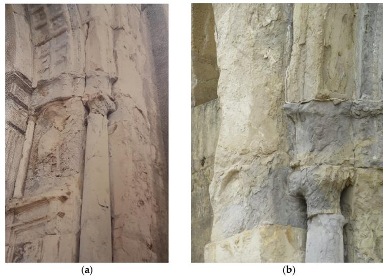
**Figure 3.** Details of different carbonate rock types and decay in the Porta Especiosa portal (a) credits: [15]; (b) credits: Alice Tavares.
