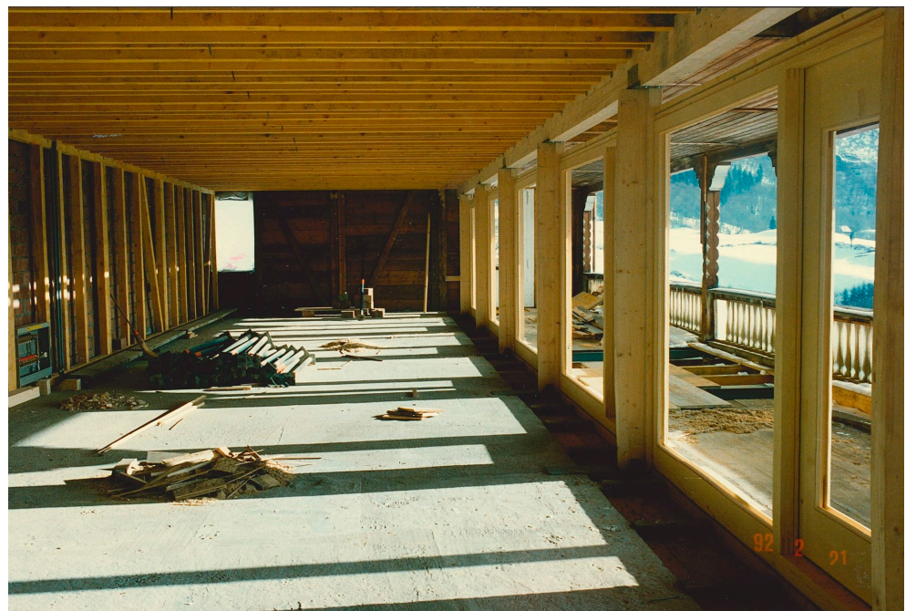
Figure 8. Walenstadtberg Housing. Timber frame construction on the second floor. Note the southwest façade featuring a glazed loggia and the entasis of the three pillars to the right. Material provided by Gody Kühnis.
