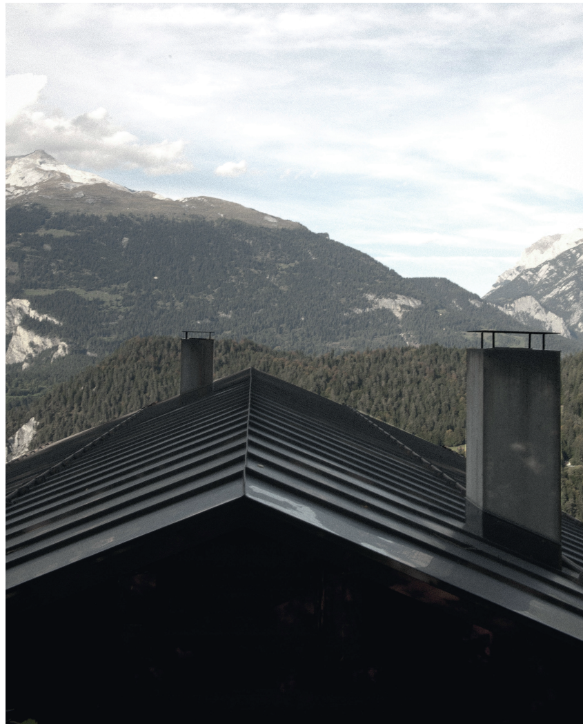
Figure 29. Gugalun House ridge from south to north. Note the original chimney in the background heating the old part and the new chimney in the foreground heating the hypocaust. Studio Adam Caruso, ETH Zurich (Simon Burri, Grégoire Farquet, Michael Fehlmann, and Lea Hottiger).
