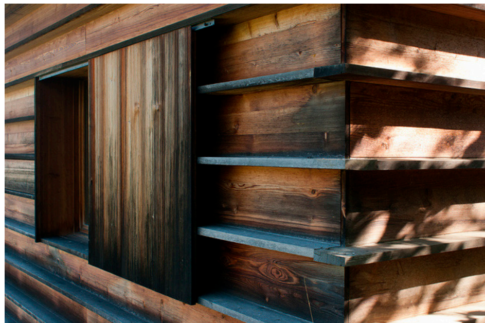
Figure 35. Gugalun House. Juts in the southwest corner that overlap the same as the old building beams. Flickr.
