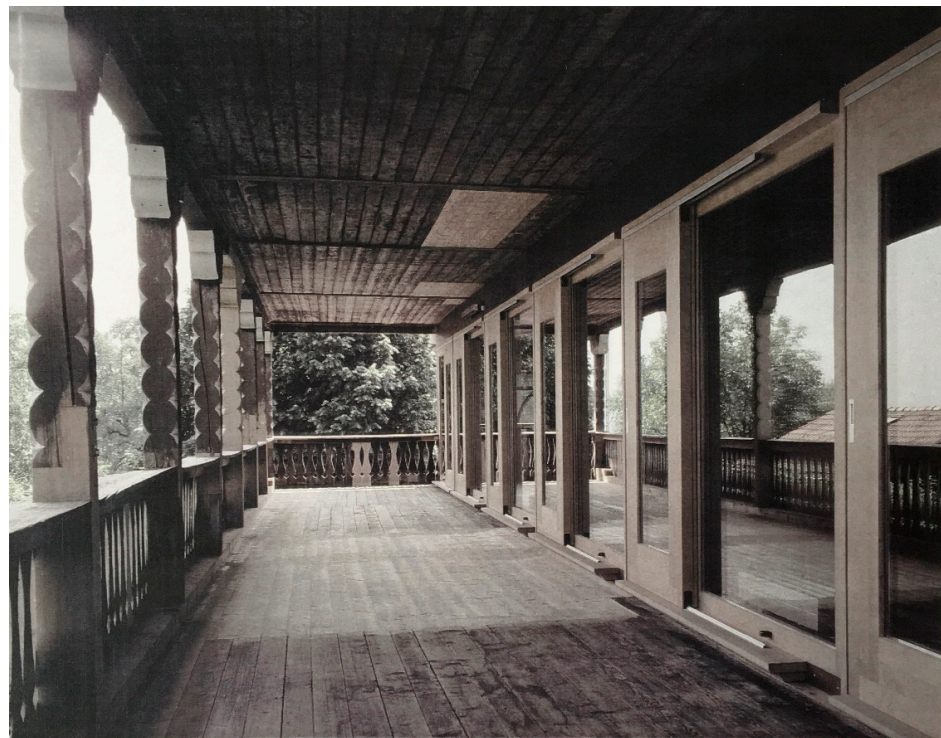
Figure 6. Walenstadtberg Housing. Veranda on the first floor. ©Peter Märkli.
