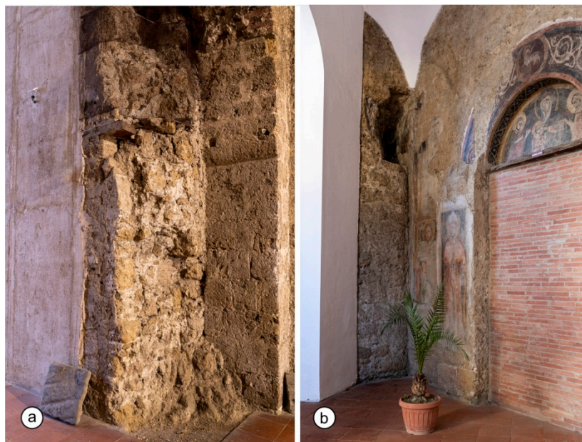
Figure 14. Examples of walls built with (a) technique “a cantieri” and (b) with technique “a bozzette” (Ph. M. Vigliotti).
