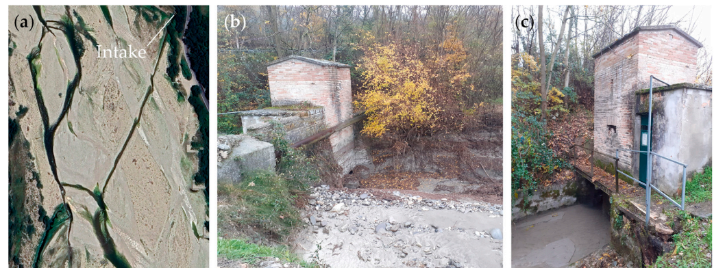
Figure 11. Intake from Parma River: (a) aerial view of the channel dug into the riverbed to allow the collection of water from the Parma River, (b) upstream view of the old intake building after a severe flood event that caused the obstruction of the system, and (c) downstream view of the intake building after the same flooding event: still water is present in the canal due to the obstruction.
