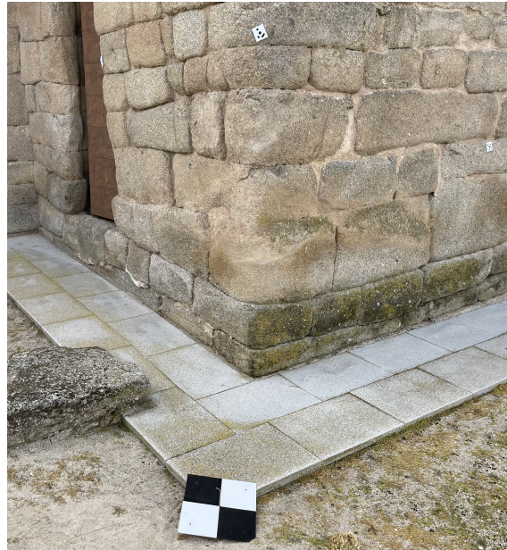
Figure 6. Target signals attached to walls and on terrain.
