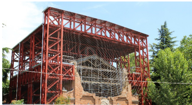
Figure 1. Church of San Luca Evangelista in Medolla (MO, Italy). Expansive metal structure to urgently secure and protect the partially collapsed masonry church. Photo credits: MiC.
