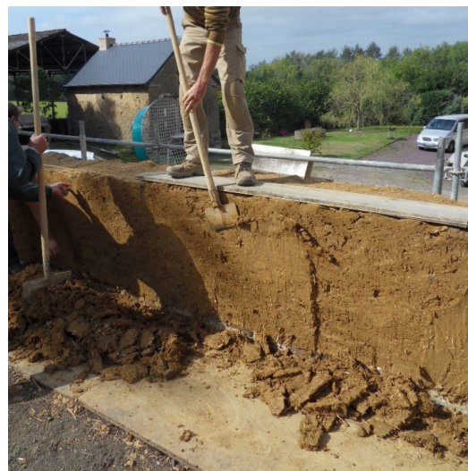
Figure 6. A cob wall in modern construction [33].
