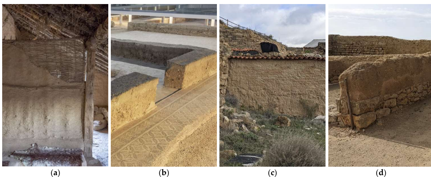
Figure 1. Groups of earthen architecture constructions identified in the study area: (a) modern reconstruction of a half-timber wall with braided reed in Numancia (Garray, Soria); (b) cob wall in the archaeological site of the Roman villa La Olmeda (Pedrosa de la Vega, Palencia); (c) adobe wall preserved in the Roman houses of B il bilis (Calatayud, Zaragoza); (d) rammed earth wall in Ampurias (La Escala, Girona).
