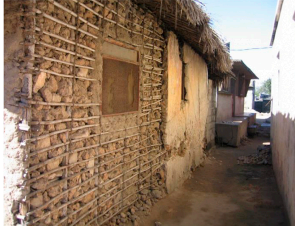
Figure 9. Photo of Macuti buildings with the wattle-and-daub structure. Reproduced from [28].
