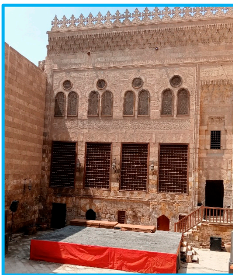
Pl. XXV: “The Maq’ad of Sultan Qānṣūh Al-Ġawrī, with aground floor includes three stores and a corridor”, 2024.
