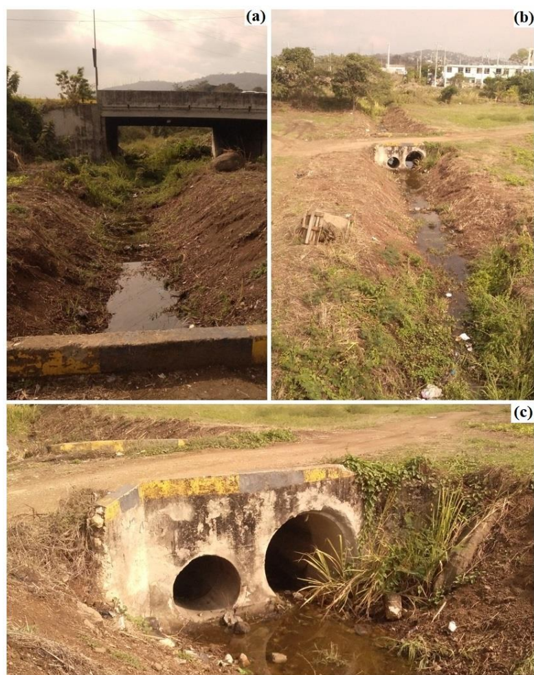
Figure 6. Identification of water dump points: (a) channel coming from the university, (b,c) connection pipes that allow the flow of water between the university and the sector called Socio-Vivienda.
