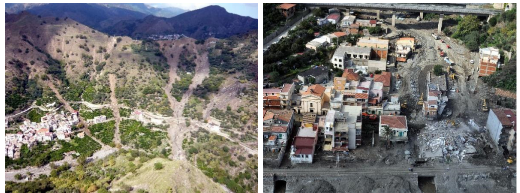
Figure 2. Damage to the infrastructures caused by the shallow landslides event that occurred in the Briga and Giampileri Villages on the 1 October 2009 and afterwards named the “Messina flood”.
