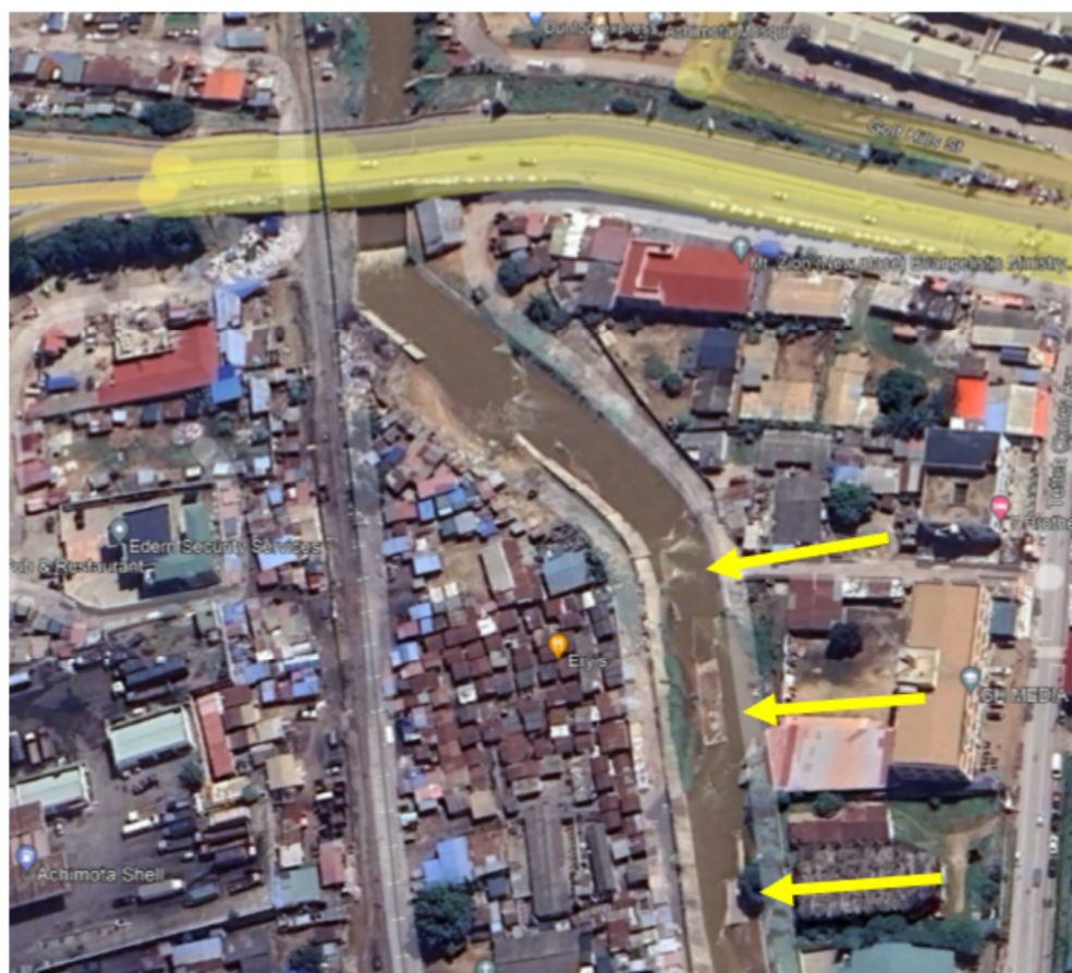
Figure 1. Collapsed concrete walls identified at the yellow arrows along the Odaw River at Achimota, 5^{\circ}37'13.0 N, 0^{\circ}13'44.5 W. Date: 6 September 2023. Source: Google Earth Pro.
