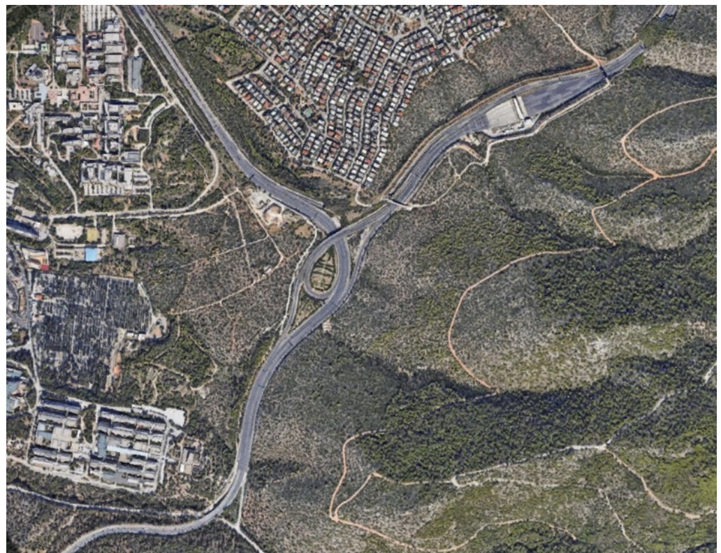
Figure 3. Example of an urban bypass motorway in an urban setting with both horizontal and vertical profiles.
