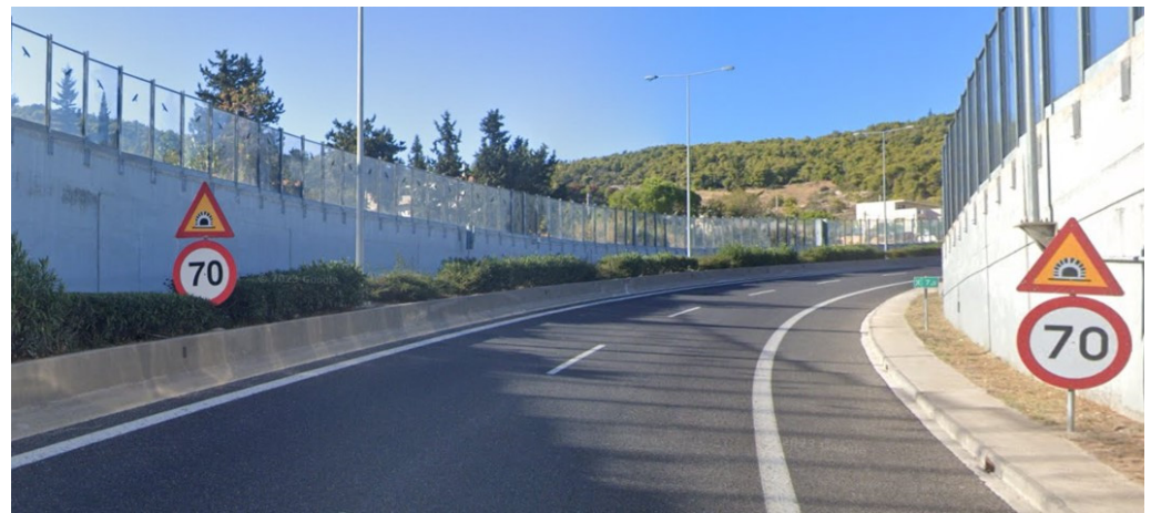
Figure 4. Example of a speed limit set on an urban bypass motorway because of its vertical and horizontal profiles.
