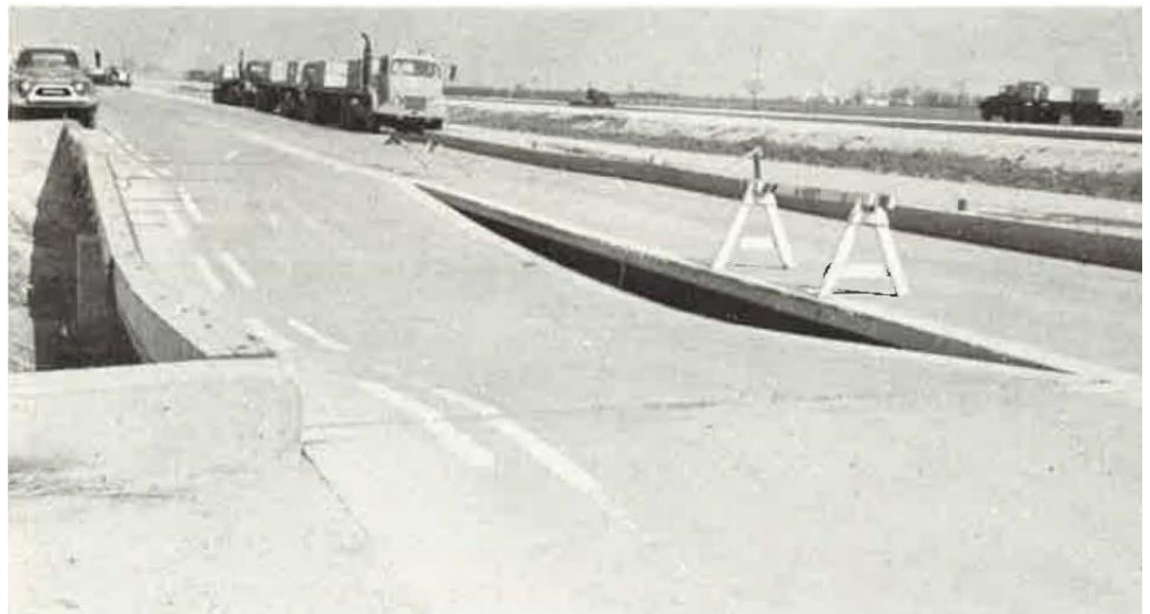
Figure 3. Bridge testing at AASHTO Road Test [21].
