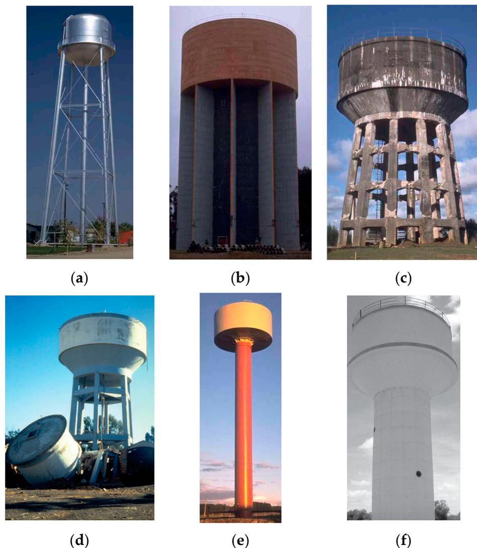
**Figure 1.** During earthquake events, a diverse array of configurations of elevated tanks sustain damage, illustrating the vast spectrum of vulnerabilities within these structures when subjected to seismic forces: (a–d) frame supports; (e,f) pile supports.
