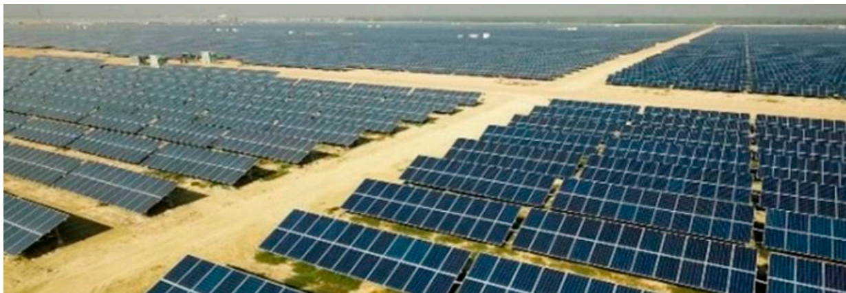
Figure 12. Quaid-e-Azam Solar Park in Pakistan [23].
