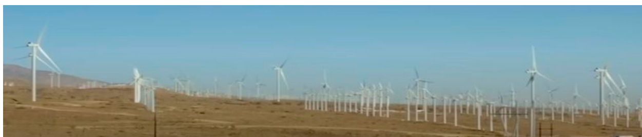
Figure 18. Horizontal axial wind turbine (VAWT) large-scale land installations [36,39].
