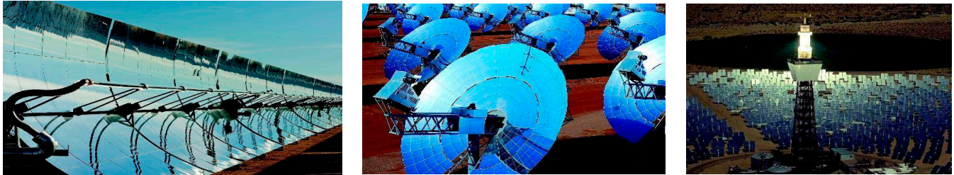
Figure 8. Various solar thermal energy collectors with concentrating mirrors [17,18].
