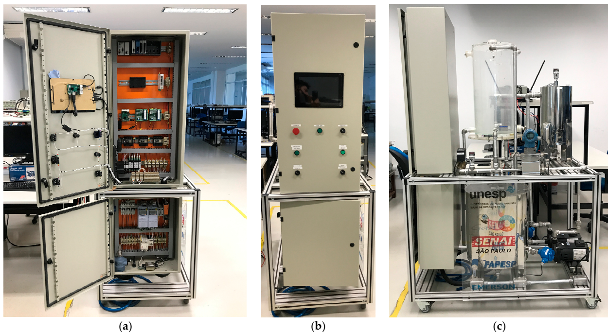
Figure 5. Industrial pilot plant: (a) Front part with open panel; (b) front part with the panel closed; (c) right side.
