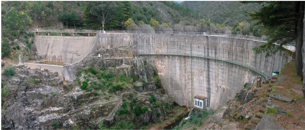
Figure 1. Downstream view of Alto Ceira dam.
