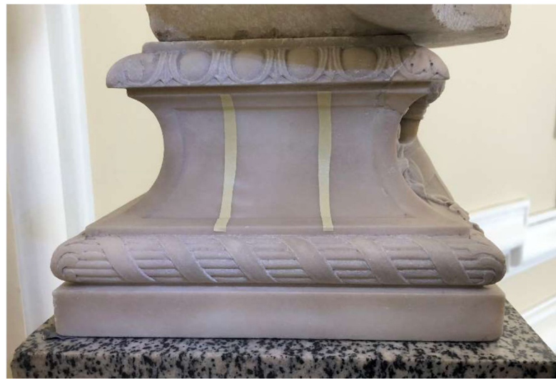
Figure 2. Cleaning areas selection and delimitation.
