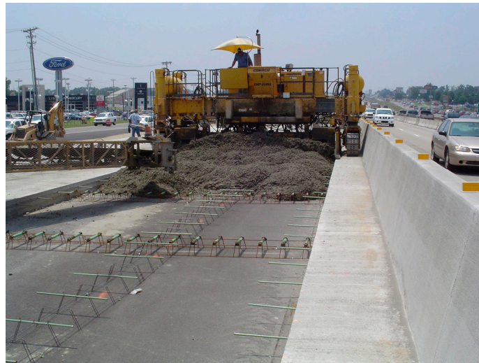
Figure 1. Typical legacy concrete pavement repair in progress.
