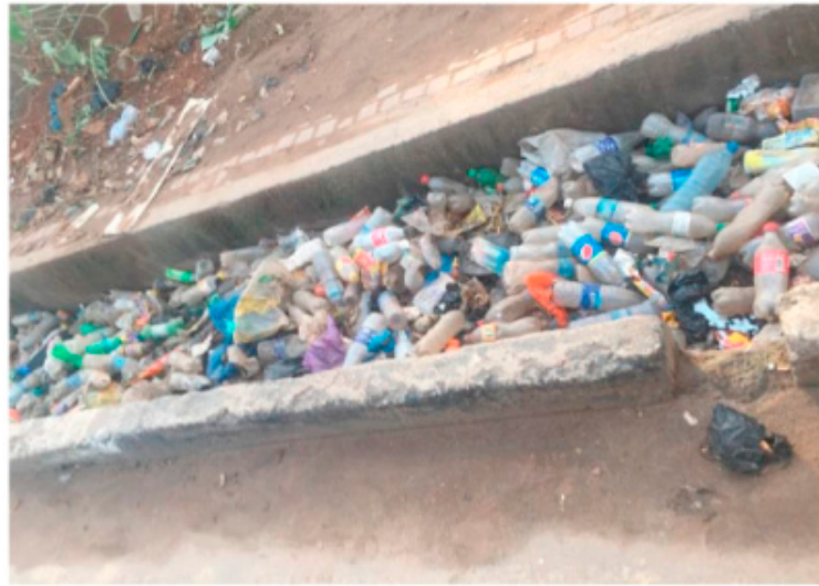
Figure 5. Plastic waste blocking drains in Nigeria [95].
