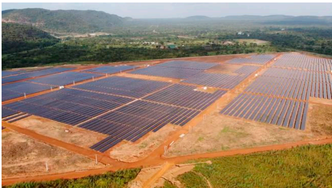
Figure 2. The 50 MW solar PV plant at Bui (location: 8.26° N, 2.25° W).
