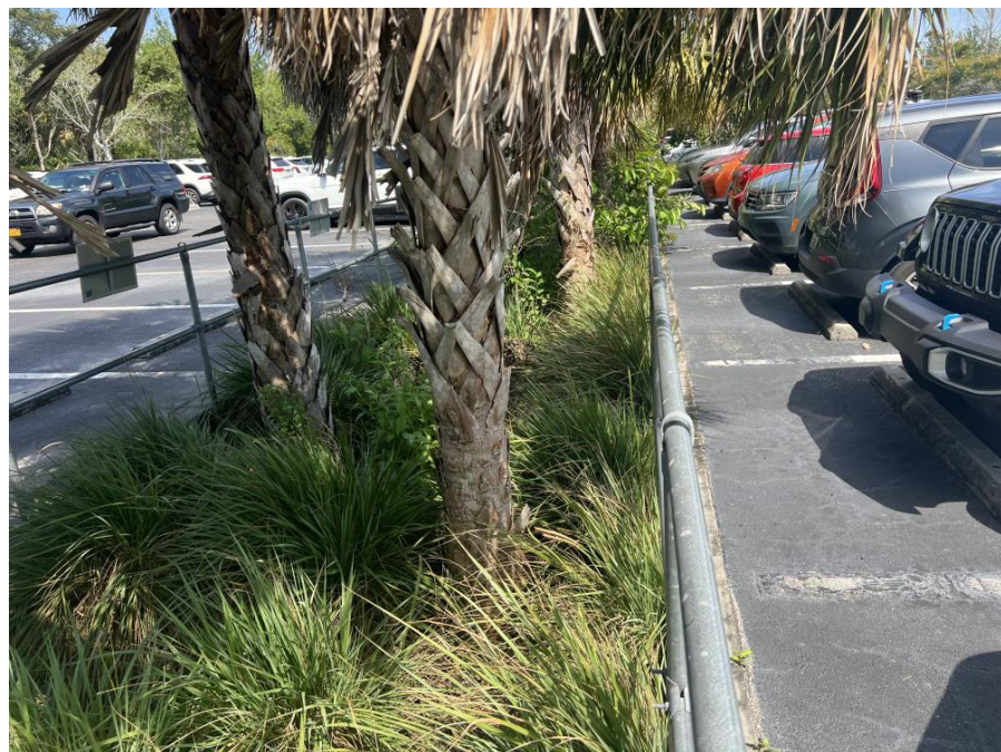
Figure 4. Bioswale dry retention wetland in the public parking area at Naples Botanical Garden, Naples, FL, USA.
