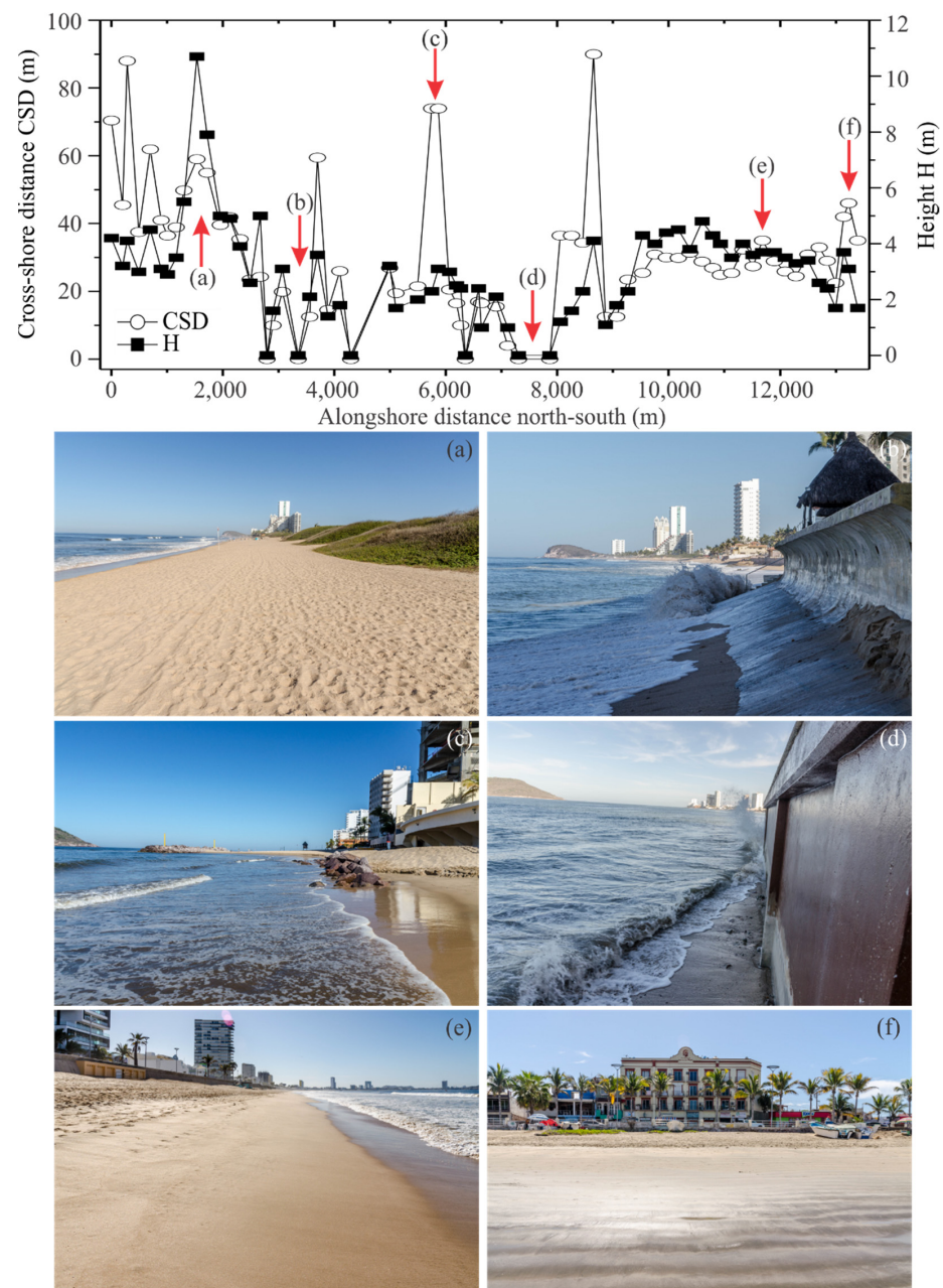
Figure 2. Field cross-shore distance and beach height along the northern section. The original conserved dune (a), seafront hotels with a hydrodynamic protective seawall (b), breakwater (c), vertical wall (d), and the concrete oceanfront corridor (e,f).
