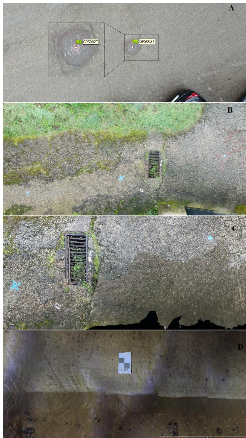
Figure 4. Examples of markers used for georeferencing the photogrammetric survey with a GNSS station in Agisoft Metashape (A), aligning lidar surveys (C) to the photogrammetric survey (B) and facilitating the alignment of the lidar survey portions of cavities (D).
