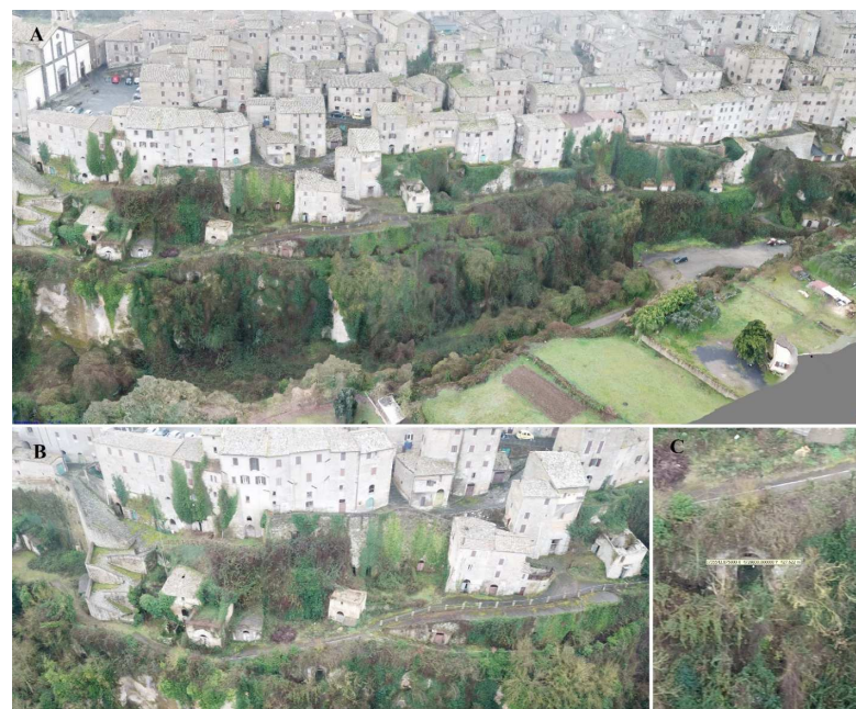
Figure 6. Textured 3D model of the north cliff of Grotte di Castro (A), photo from UAV, climbed following the photogrammetric process (B), photo detail with cavity not accessible on foot (C).
