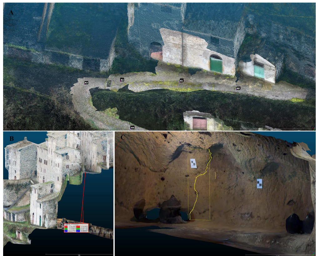
Figure 12. Examples of good alignment of the lidar model to the photogrammetric point cloud (A), use of the aligned and georeferenced 3D model to determine the geometric parameters of the cavity (B), identification in the sections of the 3D model of the rock mass joints for in-depth geostructural, geotechnical and stability checks, using the Compass plugin of Cloud Compare (C).
