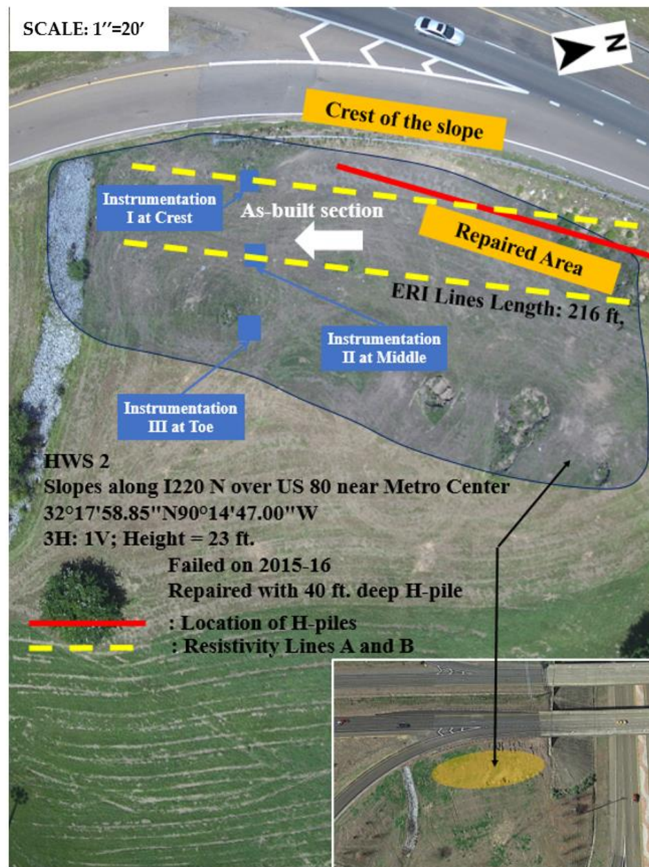
Figure 12. HWS 2 ERI and instrumentation layouts along with its characteristics (drone image-top view) (1' = 1 ft = 0.305 m).
