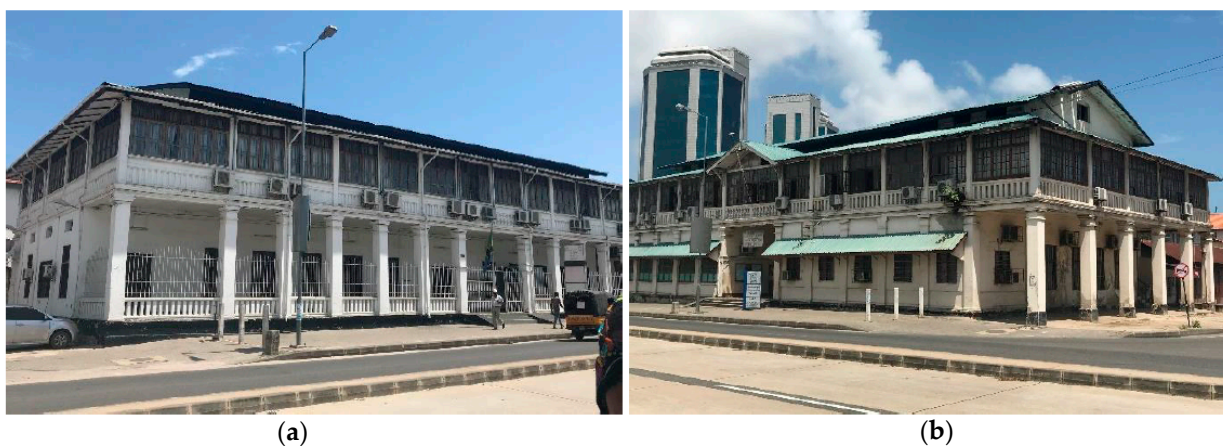
Figure 3. (a) NBS building (b) Survey and Mapping Division building; Series of German buildings with balconies covered to increase the floor plan area. (Source: Author, 2020).
