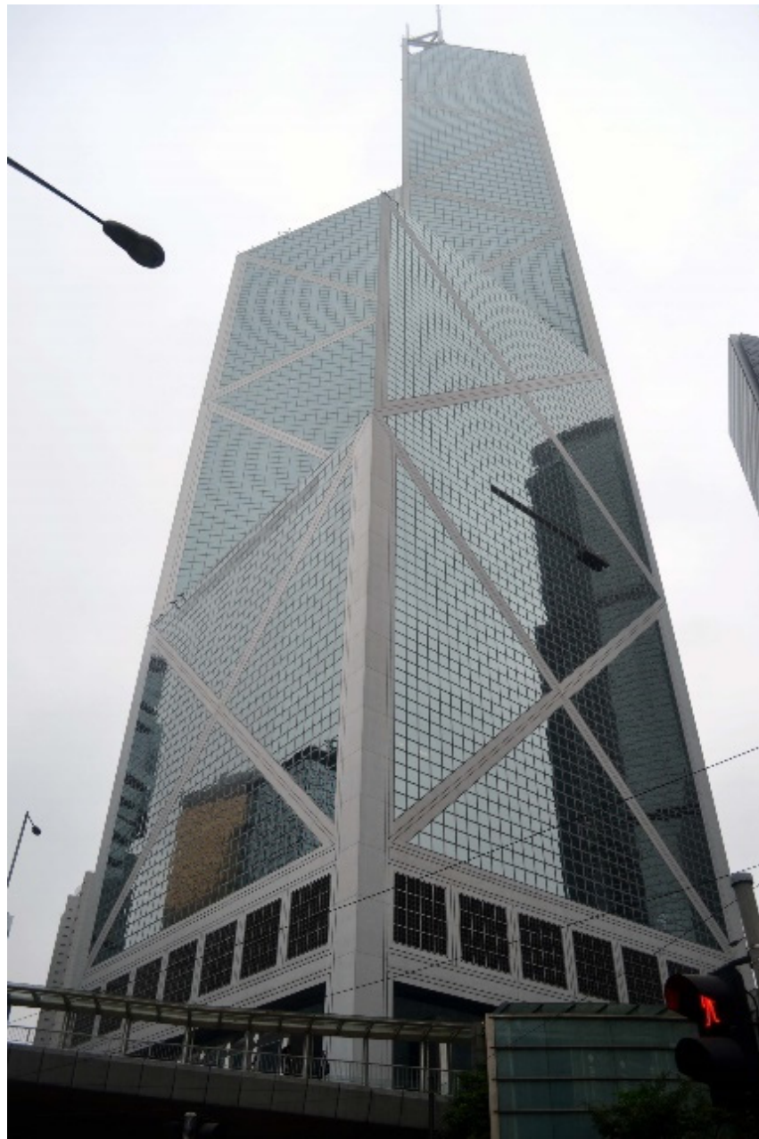
Figure 20. Bank of China Tower (1990) in Hong Kong by IMP. (Photo by K. Al-Kodmany).
