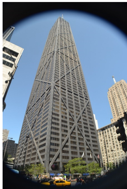
Figure 8. Braced Tube building, the John Hancock Center (1970) in Chicago. (Photo by K. Al-Kodmany).
