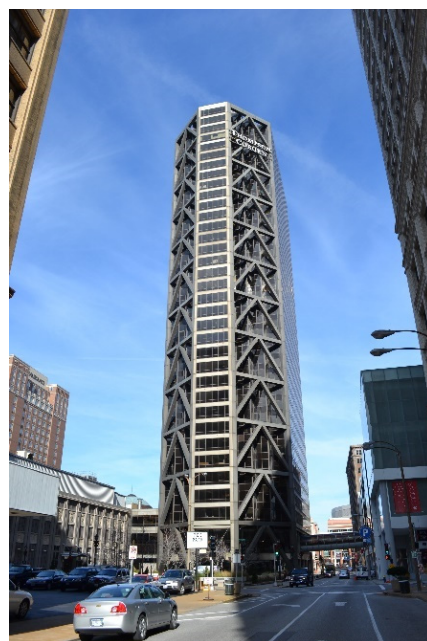
Figure 19. One US Bank Plaza (1976) in Saint Louis, Missouri. (Photo by K. Al-Kodmany).
