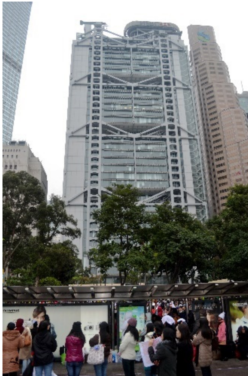
Figure 23. The Hong Kong and Shanghai Bank Corporation (HSBC) Headquarters Building (1985) in Hong Kong. (Photo by K. Al-Kodmany).
