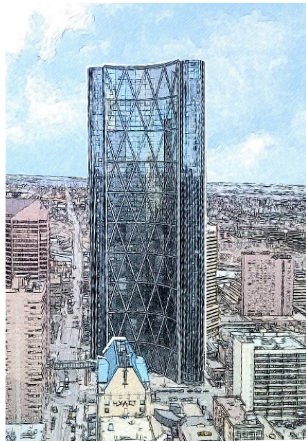
Figure 12. The Bow Tower (2012) in Calgary, Canada by Norman Foster. (Sketch by K. Al-Kodmany).
