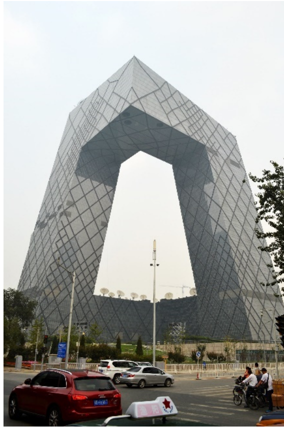
Figure 25. CCTV Building (2008) in Beijing, China by OMA. It is an example of an innovative diagrid system that improves structural performance and produces “exotic” forms. (Photo by K. Al-Kodmany).
