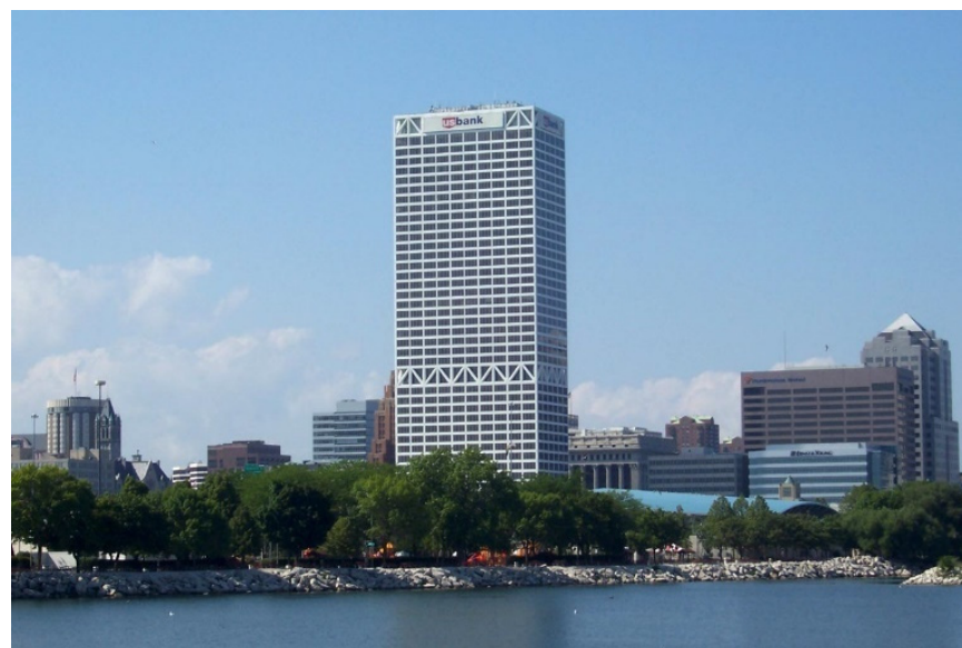
Figure 6. The US Bank (1973) in Milwaukee, WI, showing the belt trusses. (Source: Wikipedia).
