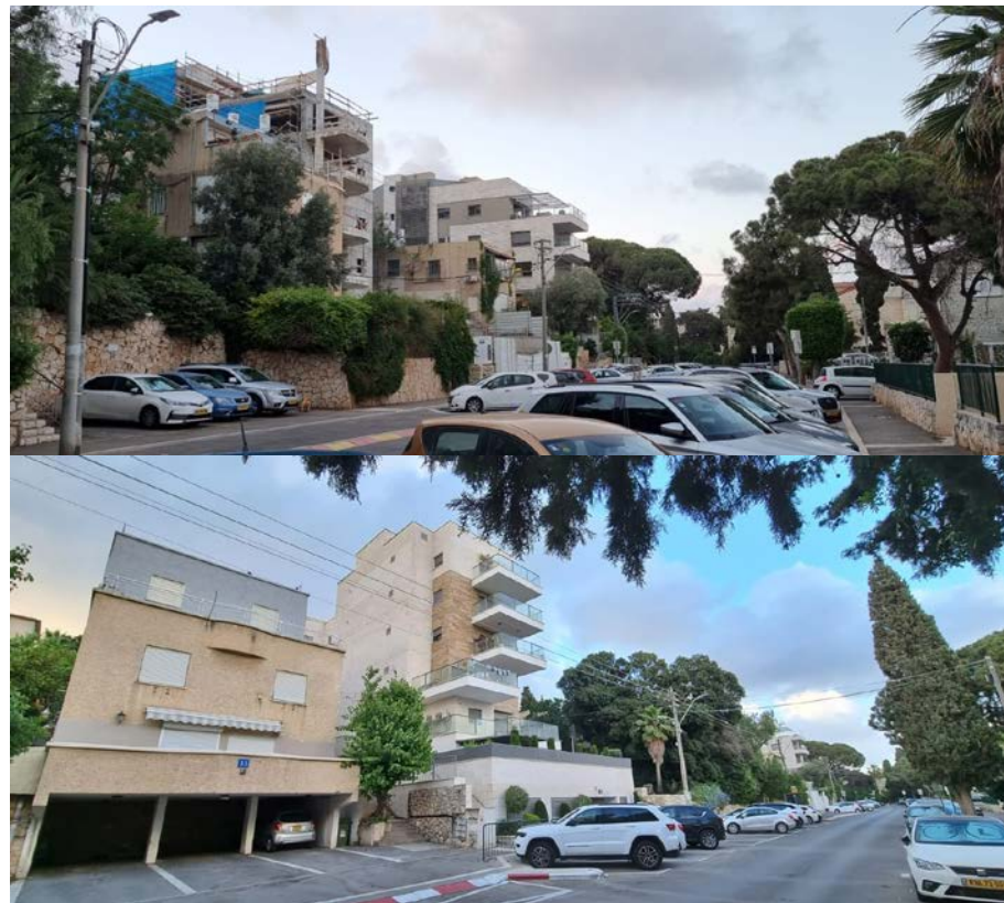
Figure 7. De-Israeli site, during the transformation of TAMA38 construction. A view from the inner side of the site. Photographed by the author, 2022.
