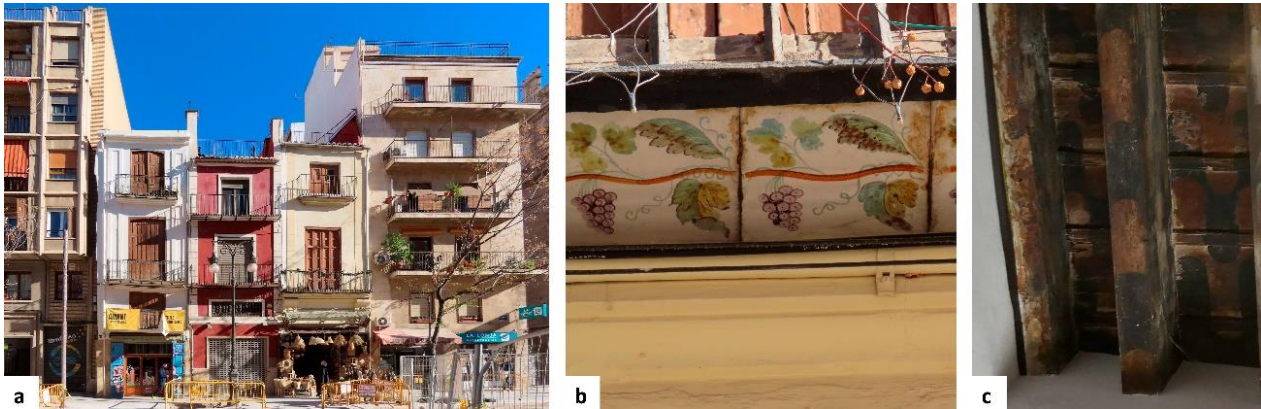
Figure 18. (a) Buildings on the stretch from the market square between the Lonja and Tabla de Cambios; (b) detail of a balcony from the mid-18th century; (c) ceiling with wooden beams, laths and ceramic tile that could be dated to the 15th century. (Source: authors).
