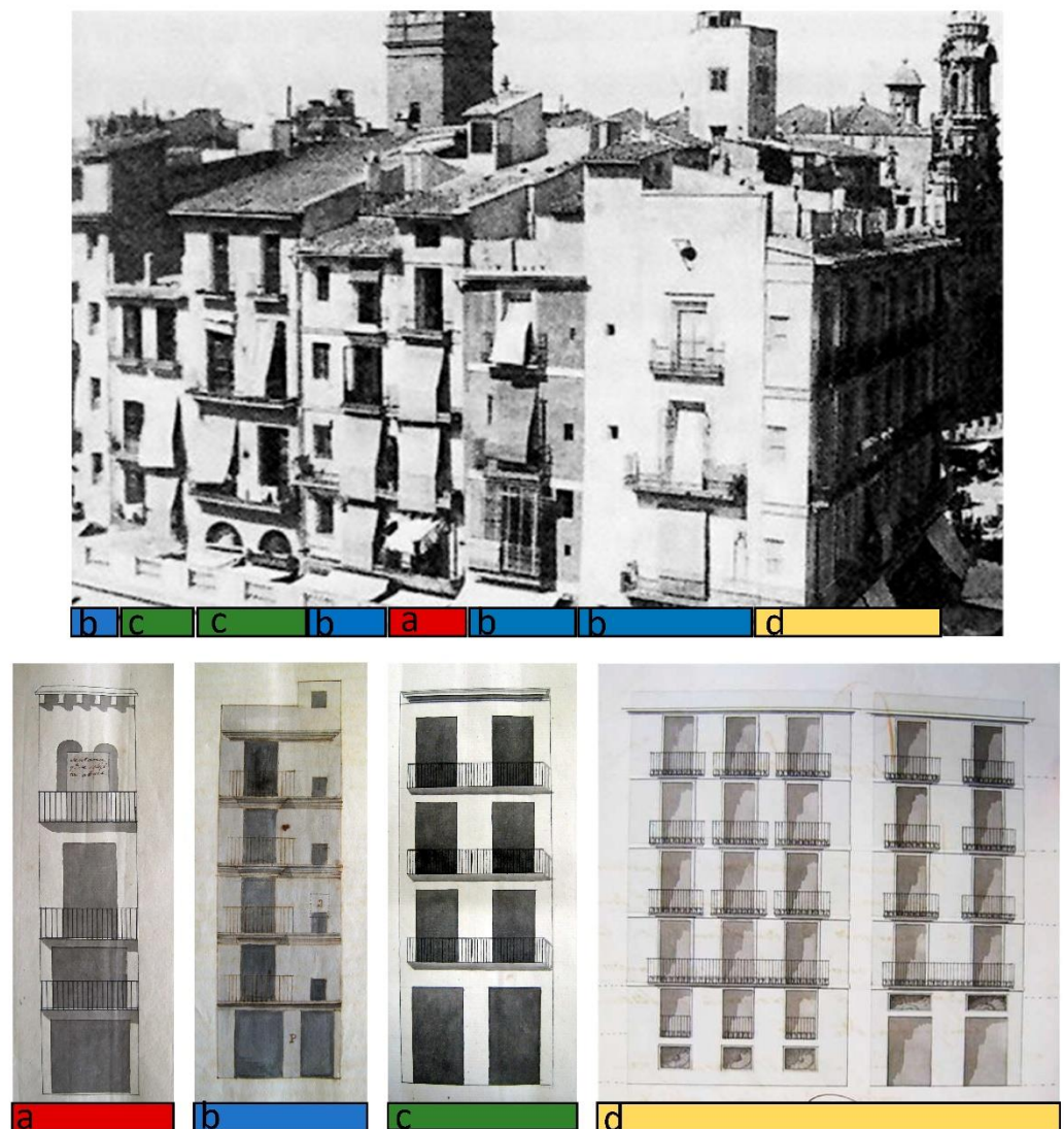
Figure 17. In the upper part, a photograph from the beginning of the 20th century where the different types of houses in the market area can be recognised; in the lower part, four drawings from the Historic Archive of Valencia that illustrate the different types of houses: (a) workshop dwellings (1793); (b) stairway houses (1794); (c) workshop dwelling with a double shop window (1796); (d) communal residential buildings (1854).
