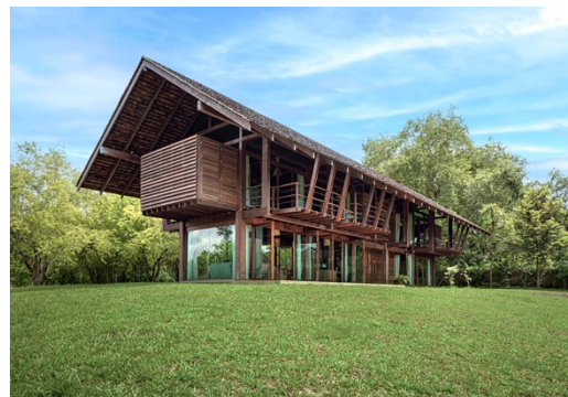
Figure 2. So too can the built anticipation of intense sun and rain in the form of an enveloping roof canopy (image source: PAVA Architects).
