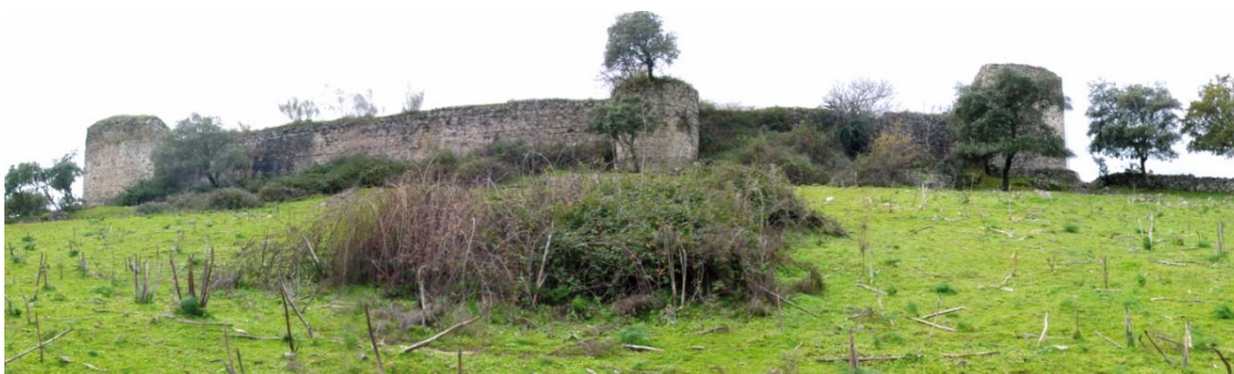
Figure 8. Northeast elevation, before the rehabilitation of the BIC, year 2000.
