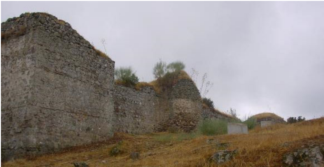
Figure 3. Initial state, before the architectural intervention.
