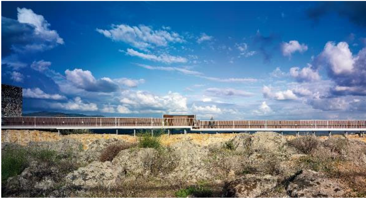
Figure 7. Photograph of the catwalk, 2012.
