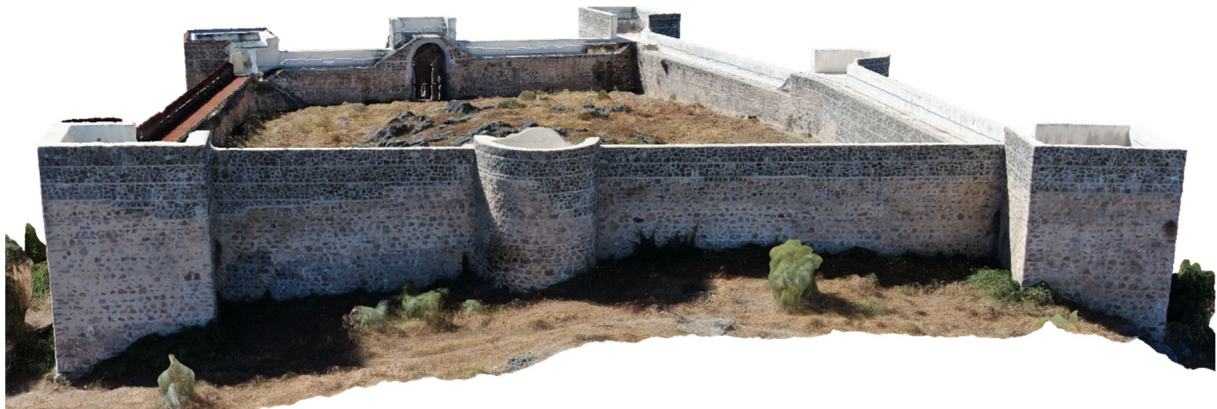
Figure 19. Northwest elevation; image obtained from the photogrammetric process, 2020.
